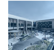
City Center Almaza - LEED GOLD Certification
