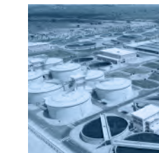
Gabal Al Asfar Wastewater Treatment Plant
