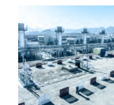
GE LM6000 at Sharm El Sheikh Power Plant
