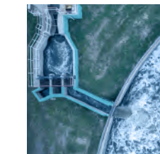
Madinah 3 Independent Sewage Treatment Plant
