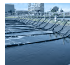
Activated Sludge Plant – Germany
