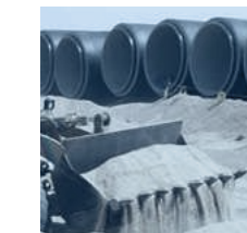
6th of October Water Transmission Line
