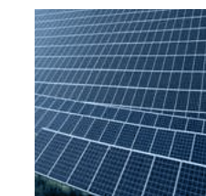
Sharm El-Sheikh Solar Power Plant
