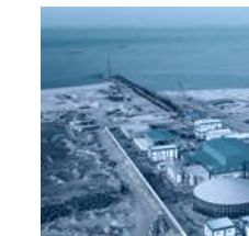
New Mansoura Desalination Plant
