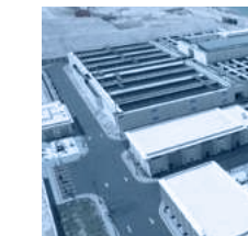
Mahsama Water Treatment Plant
