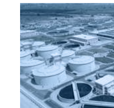
Gabal Al Asfar Wastewater Treatment Plant
